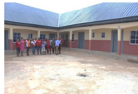
New staff quarters at Uloanwu, with ten self contained units
