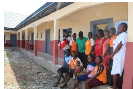
Uloanwu staff quarters with 10 self contained units
