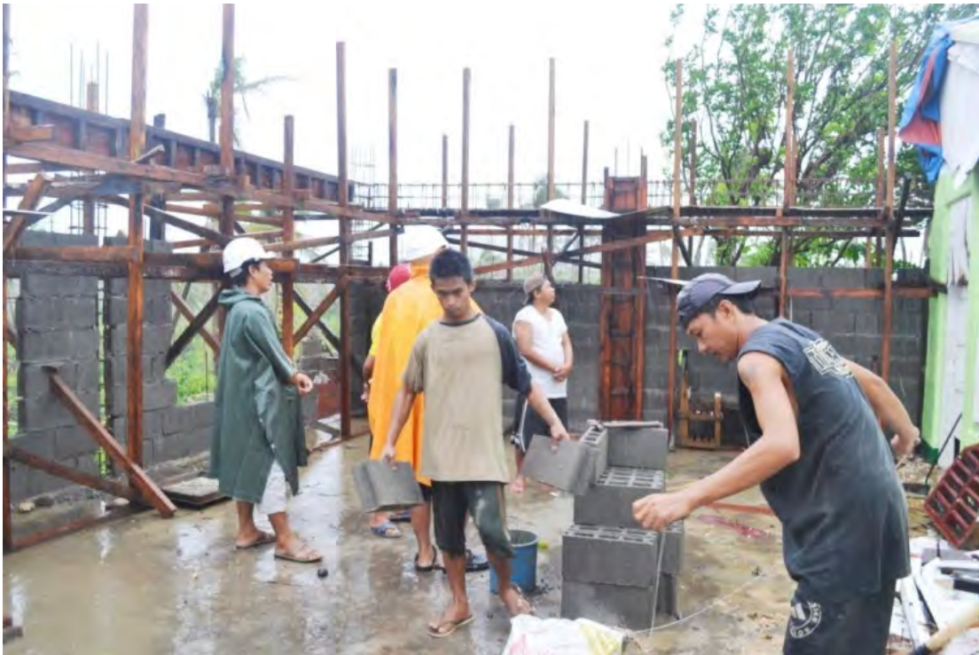
Construction work in building 6
